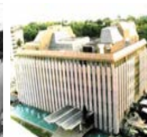
The renovated building, Dar es Salaam, 1989
