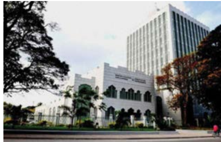
Bank of Tanzania's Zanzibar branch office building (2004)
