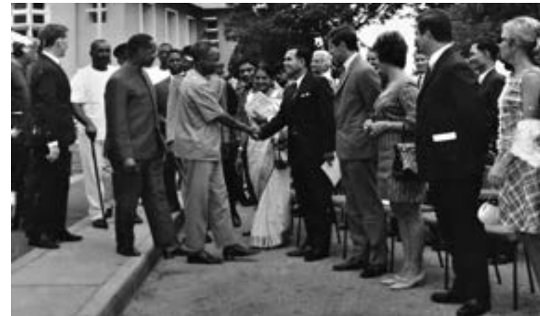
Mwalimu Nyerere shaking hands with the contractor of the Bank's first headquarters building on 9 th December 1966. Others in the photo include the first President of the Revolutionary Government of Zanzibar, Mr. Abeid Amani Karume (holding a walking stick) and the first Bank of Tanzania Governor, Mr. Edwin Mtei (on the right hand side of Mwalimu Nyerere).
